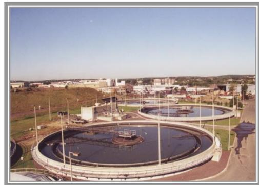
The secondary treatment facilities are comprised of Oxygenation Tanks, Pure Oxygen Generating Plant, Liquid Oxygen Storage Tanks, Secondary Clarifiers, Return Sludge Pumping Station and Splitter Box, Sludge Thickeners, Pumping Station, Sludge and the Dewatering Building Addition.
